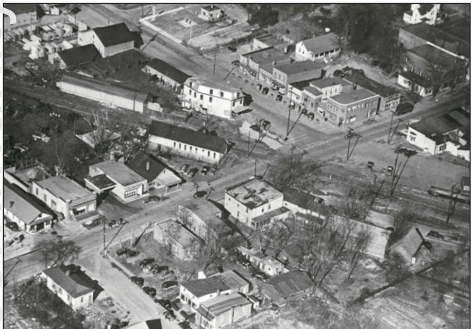
East Falls Church- Lee Highway and Fairfax Drive, 1946
