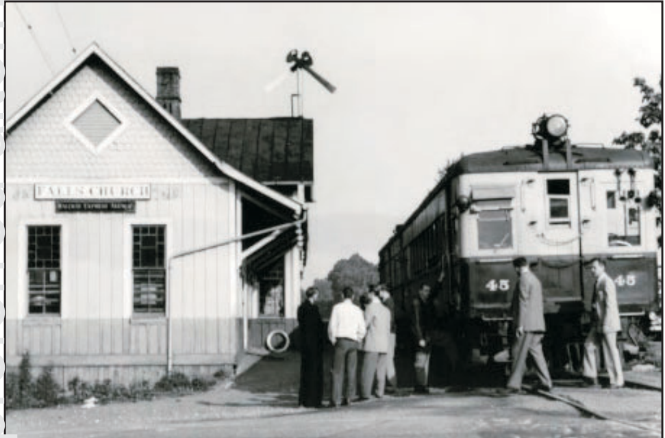
East Falls Church Trolley and Station
